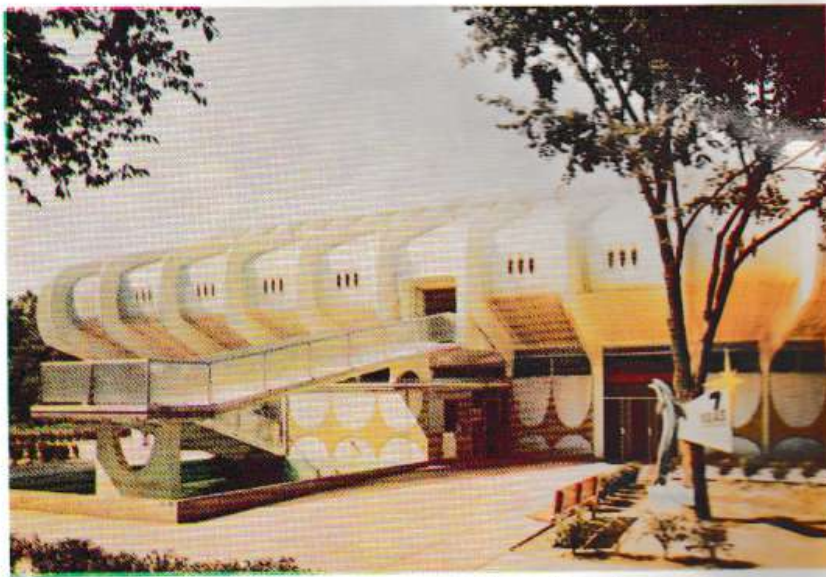
Entrance of the Seven Seas Panorama of Brookfield Zoo, Brookfield, Ill. Note Plexiglas door which is built in sections and can be removed during the summer months.
