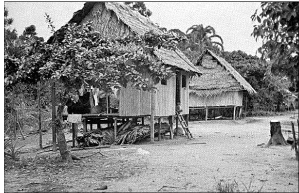
The houses of the Ticunas are up on stilts to keep them dry when the Amazon overflows its banks.
